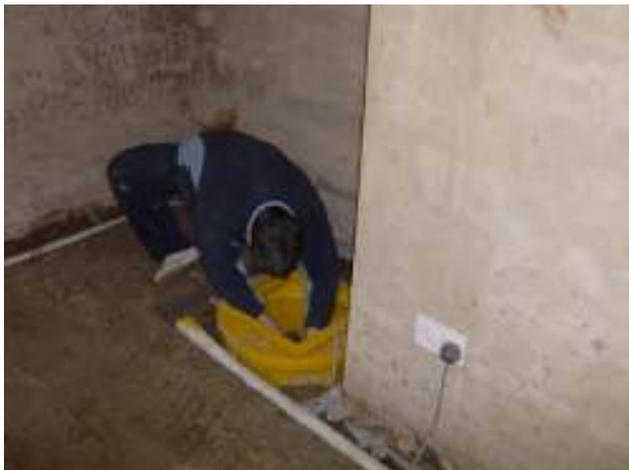
Sinking the sump into the floor and fitting the pump
