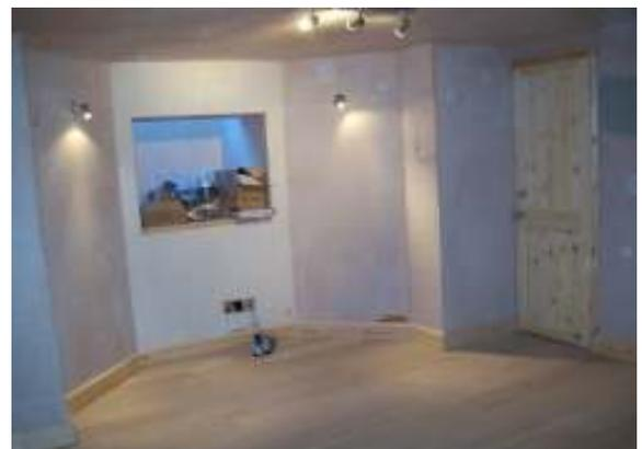
Second fix electrics are in progress and skirting boards have been fitted
