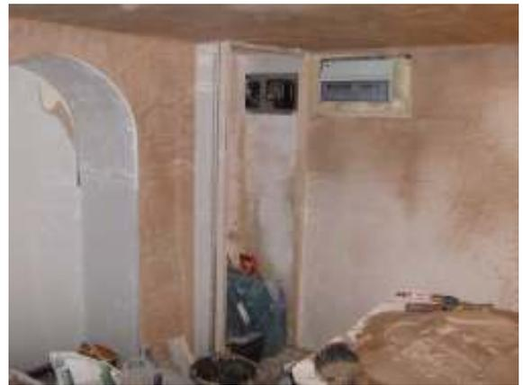
Plasterboard has been applied to the stud work and a finishing coat of plaster is being applied
