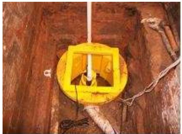
In some cases it may be advisable to install a second back-up pump within the sump. This gives added security in case of primary pump break down.
