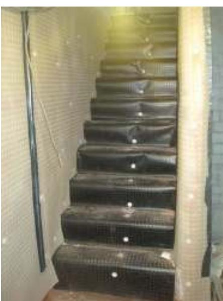
the full range of dampness issues found in cellars and basements from flooding to general dampness or problems with surface salts. As well as being completely waterproof the membranes are impervious to salts present in the groundwater guarding internal decorated surfaces from staining. Other uses of these membranes include turf covered roofs and barn conversions.
