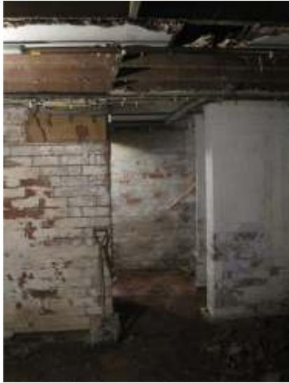
Digging out the floor to gain a few extra inches of head height
