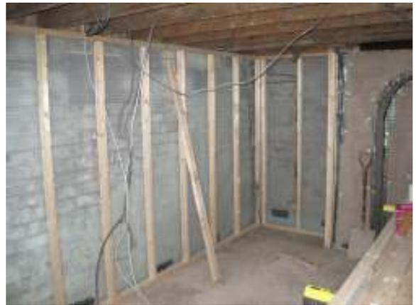
Stud work is erected over the membrane so that insulation can be incorporated
