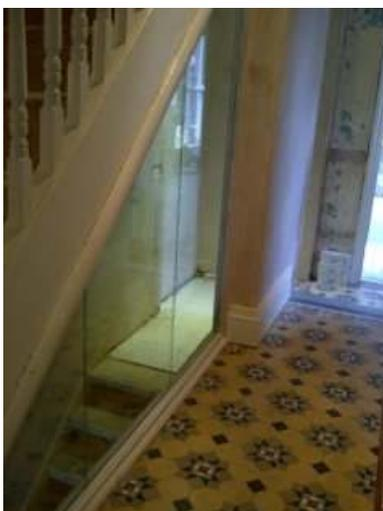
A glass panel installed at the top of stairs to throw more light onto the stairs leading into the newly converted room
